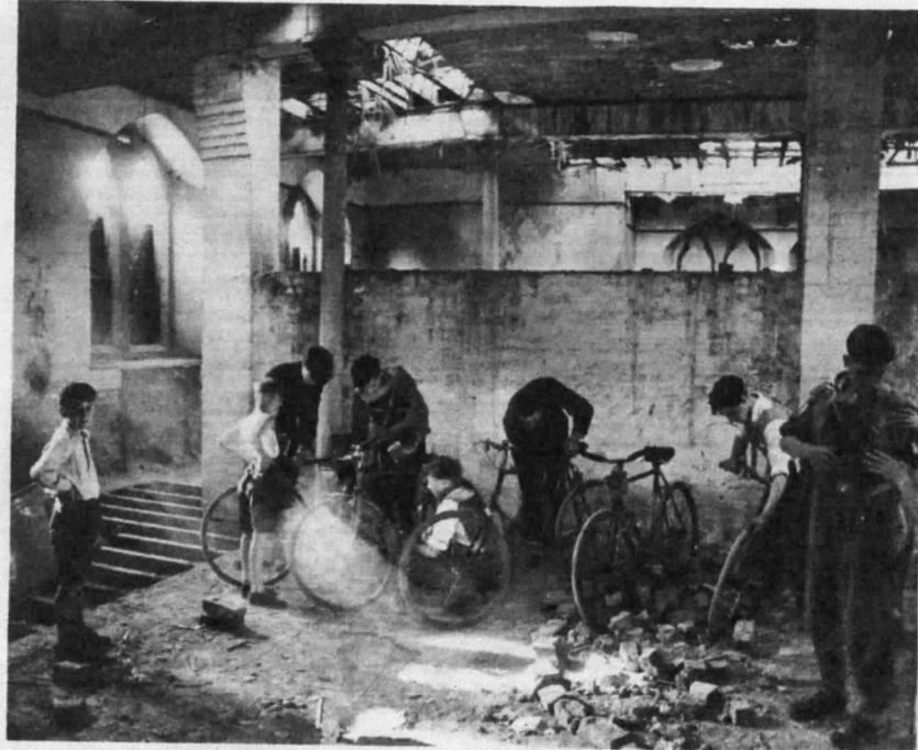
'In the Pits': They Were Once a Methodist Chapel Before it was bombed they used to come here to Sunday School. Now New Cross youths who have established a cycle track on the adjacent bomb-site, use it as a dressing-room.
